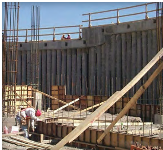
Earth Retention Wall Design and Construction
