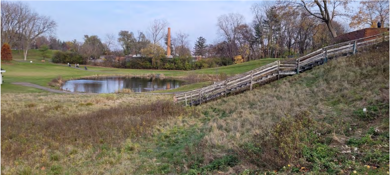
View East of Staircase
